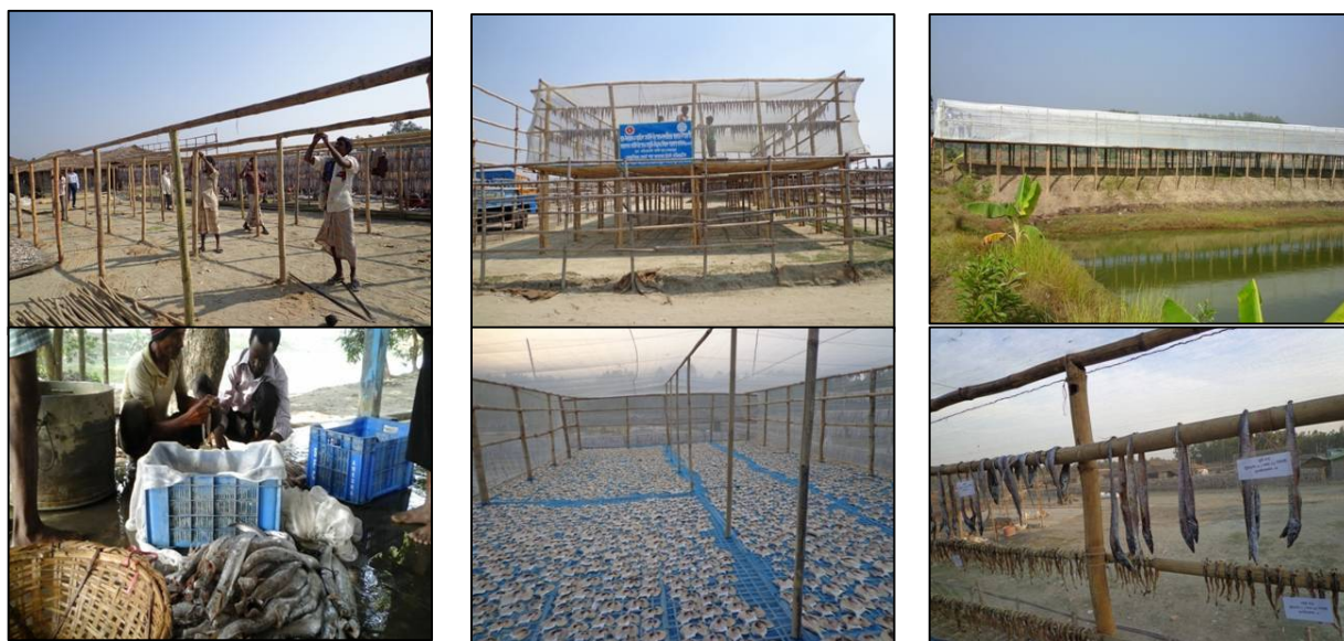
Fig 1. Construction improved traditional fish drying facilities suitable for large scale entrepreneurs.
